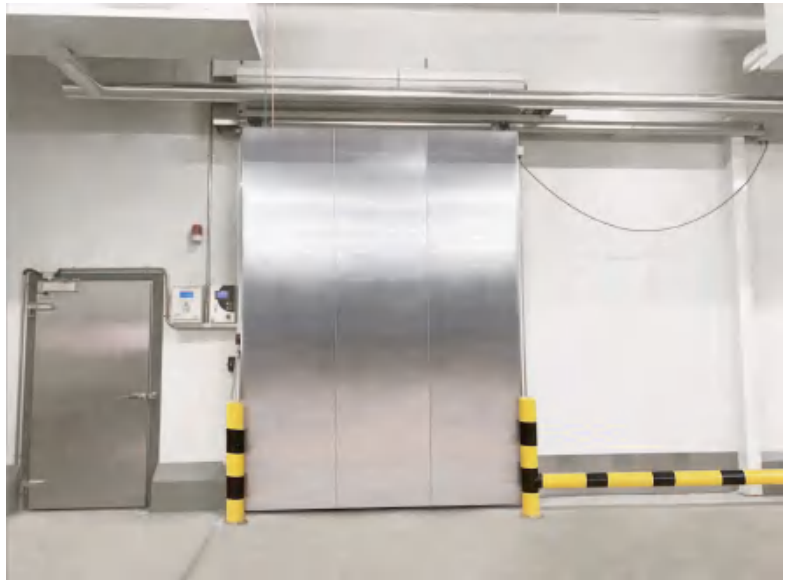
Cold Storage Doors
